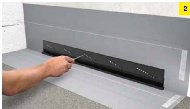
2 Thanks to the height-adjustability of the tiling aid, the drainage slot can be set to exactly 20 mm.
