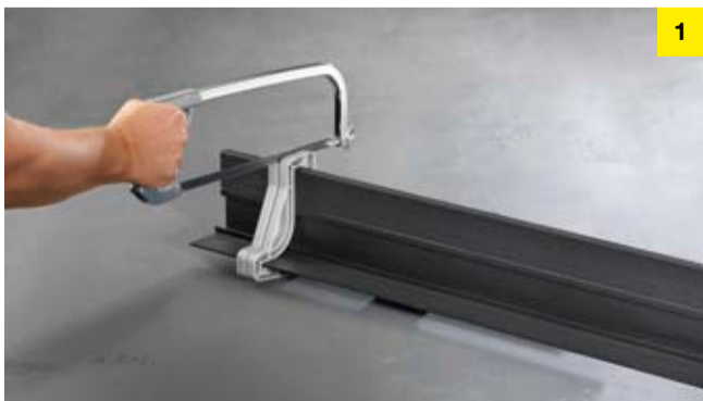
1 Shorten the channel base unit with a hacksaw and the cutting aid, deburr cut surfaces, apply sealing caps and screw tight.
