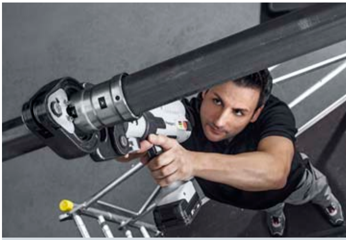
Quick, simple and safe assembly without any welding.
