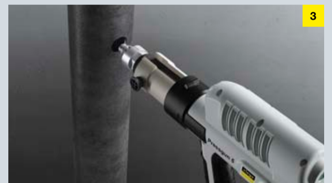
3 Press the press-in connection into the pipe with the press machine and press insert.
