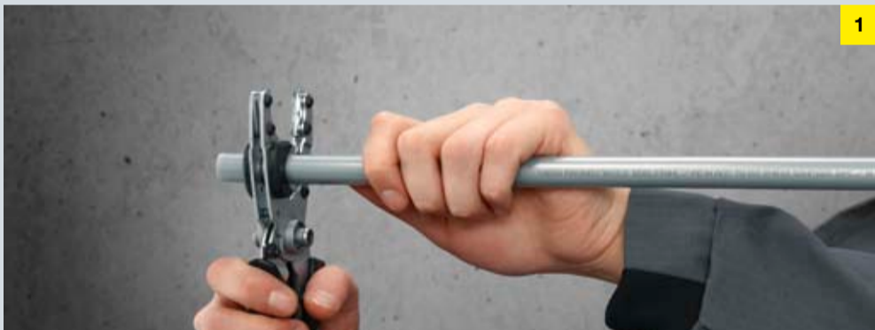
1 Cut pipe to length using the Raxinox pipe shears.
